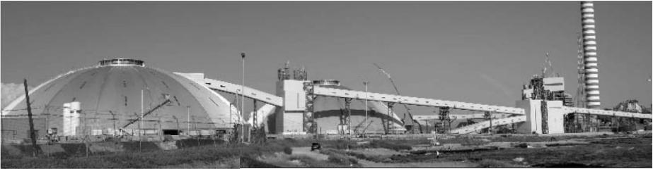
Figure 1. Transport and storage system for coal
