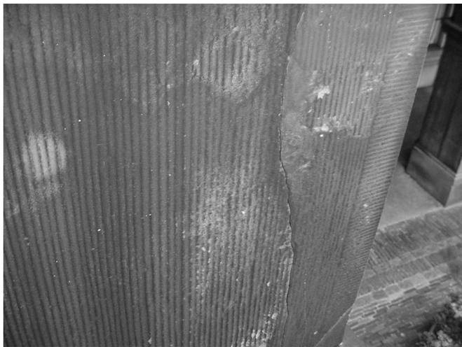
*Figure 3: Example of black weathered Obernkirchen sandstone on the façade of the Staten-Generaal, The Hague (january 2003)*
