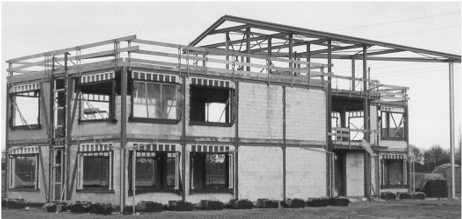
*Figure 1: Infilled frames - beams and columns confining walls*
