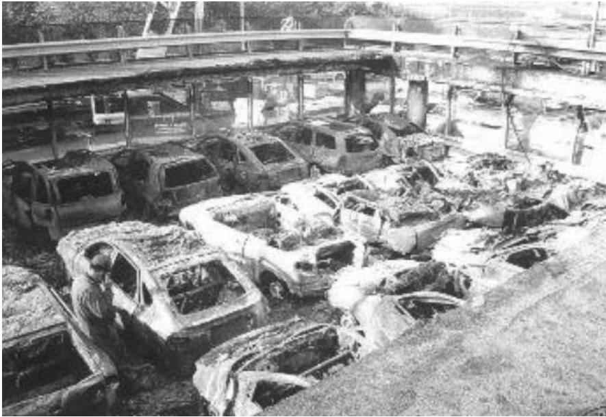
Figure 1. Picture after the fire in the car park near Schiphol airport (picture from [1])
